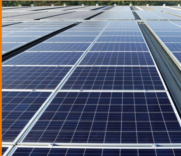
JREDA Government Building, Jharkhand
