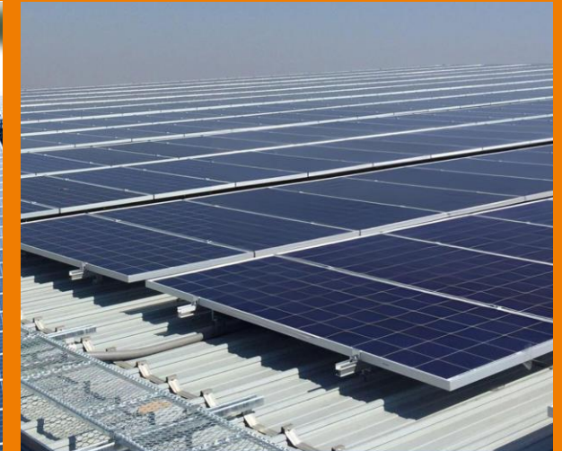
Shavya Geotex, Tadkeshwar
