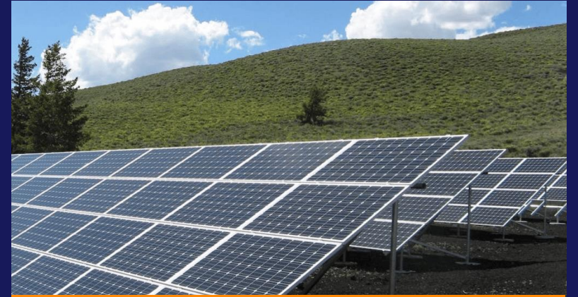
Solar Power Plant
